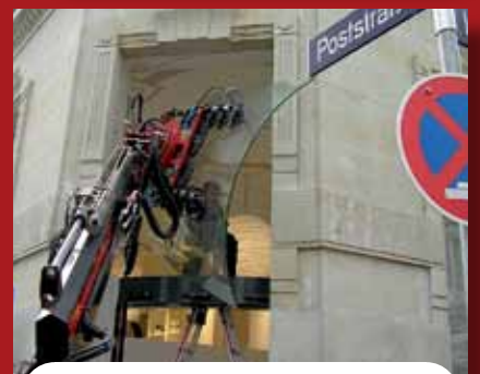
Glass suction cup, spherical
