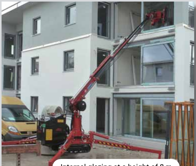
Internal glazing at a height of 8 m
