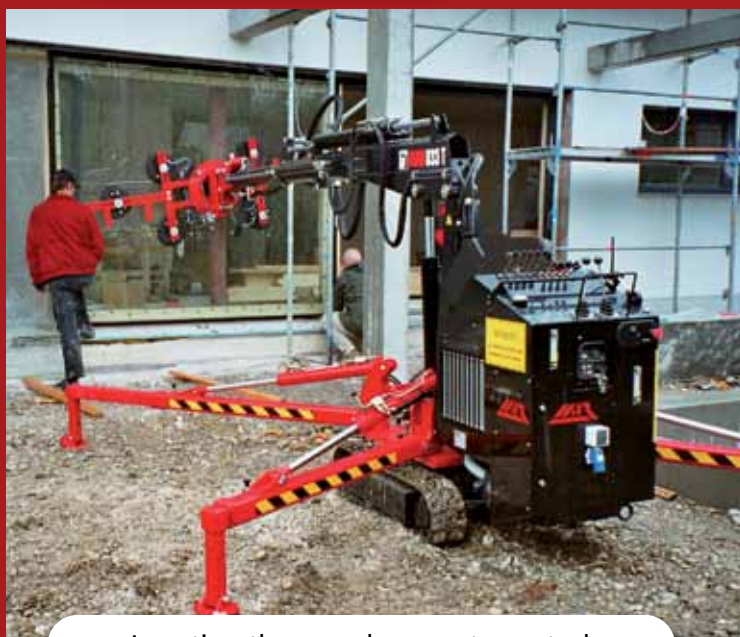
Inserting the pane by remote control
